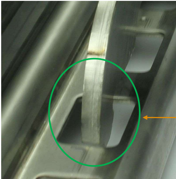
Correct position of the brake in the Frigowall track
